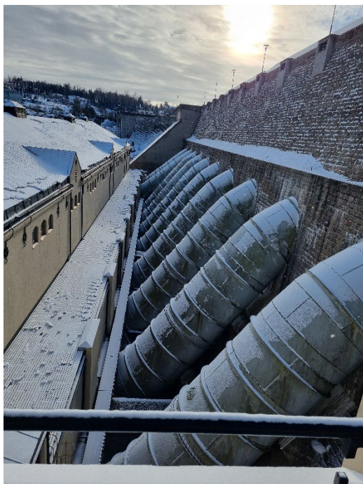
Picture 1 (left): Penstocks leading water into the hydropower station
